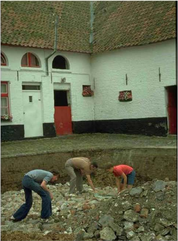
Father and sons separating the re-usable bricks from the rubble. Picture taken at a farm around 1970.
