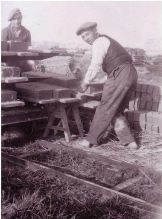
Stacking stones after they were baked in a field oven. (1920)
